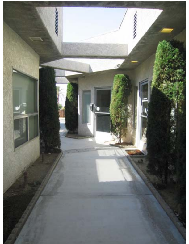
Interior courtyard entrances
