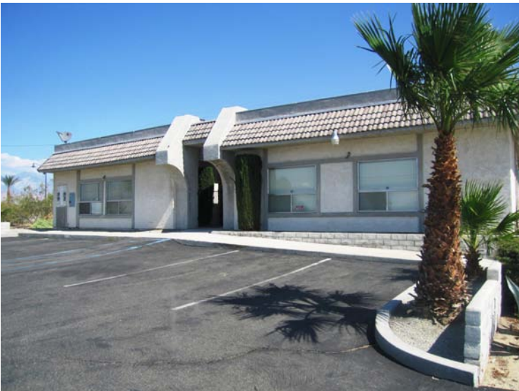
Back side of building.
